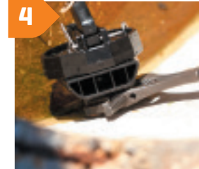
Valve body is suitable for final tightening with a wrench/multigrips to ensure valve is perpendicular.
