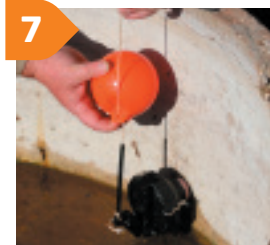
Check float position against side of trough.
