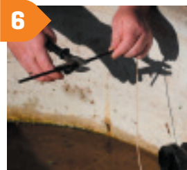
Trim the anti-tangle tube if required and secure loose end of cord to float.
